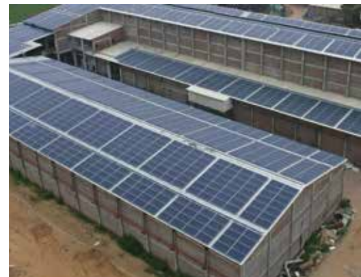
Chandpur Enterprises, Bijnor Capacity 851 kW
