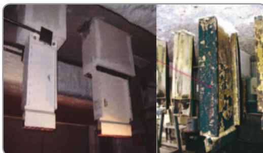
Fire barrier test
